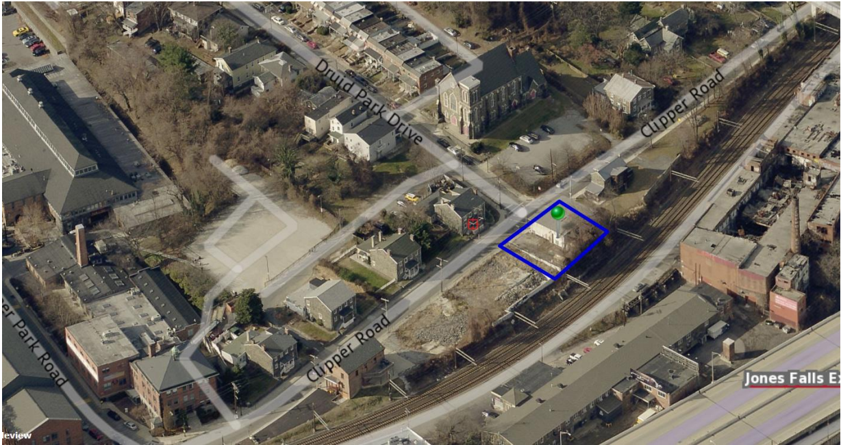
Image 3: 3535 Clipper Road site – Aerial view from southeast, December 8, 2019
