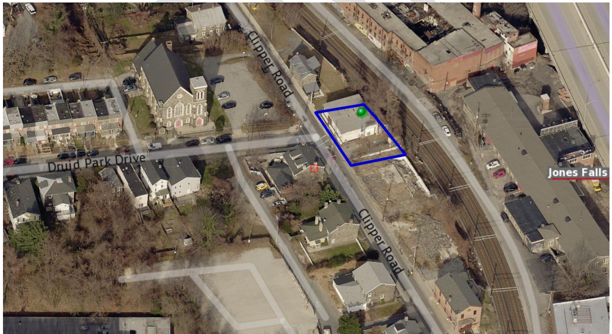
Image 2 : 3535 Clipper Road site – Aerial view from south, December 8, 2019
